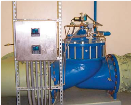
Modulating Level Control with Metering
