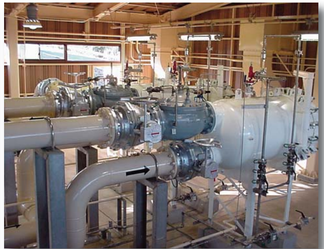
Filter and Flow Control
