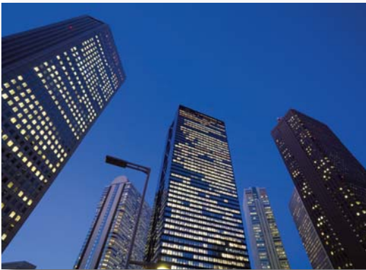
Commercial High-Rise Fire Protection: Breach Control, Pressure Reducing, Pressure Increasing, Fire Pump Control, Pump Check and Air Release
