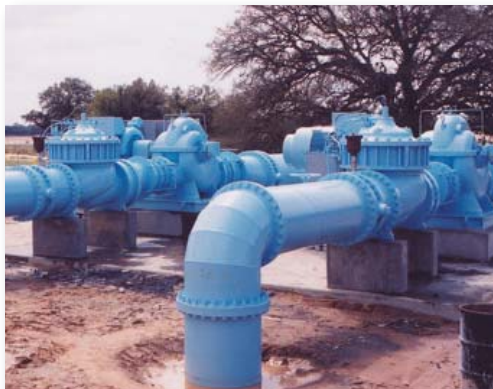
30-Inch Pump Control Valves
