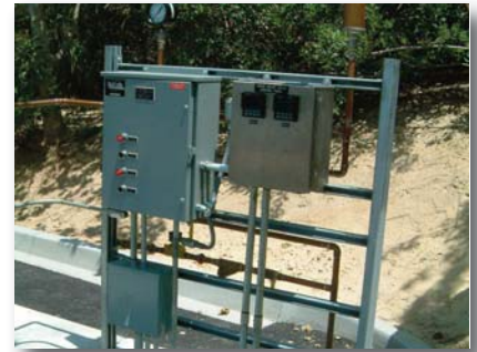
Remote SCADA control
